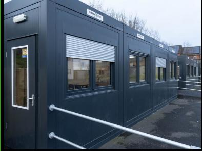
The 16 CTX modules were manufactured offsite with our plug and play system, meaning only a matter of a week for connections on-site. Our team worked successfully to complete the additional teaching space accommodation to avoid disrupting the start of the new school year.
